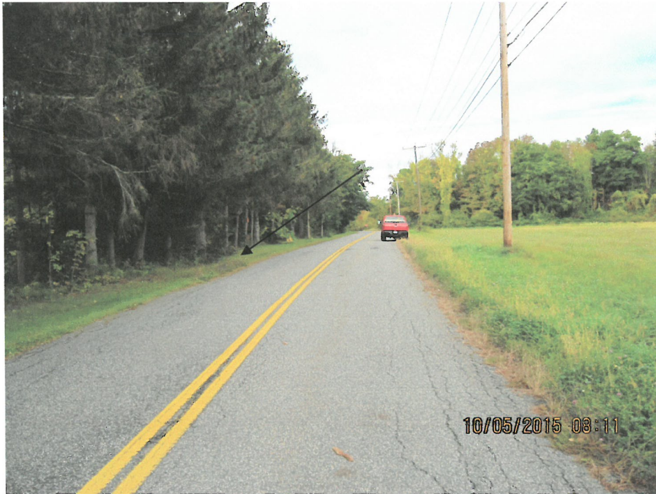
41 West Plain Rd Looking West
